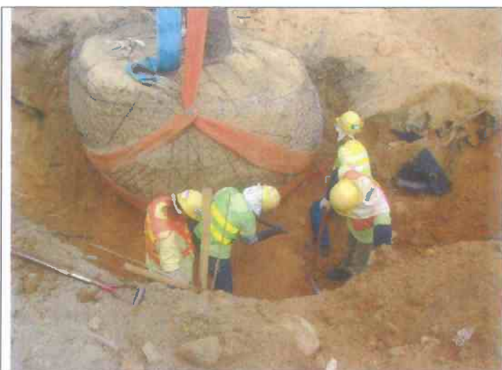
Figure 3 Root ball installed with chain link fence
